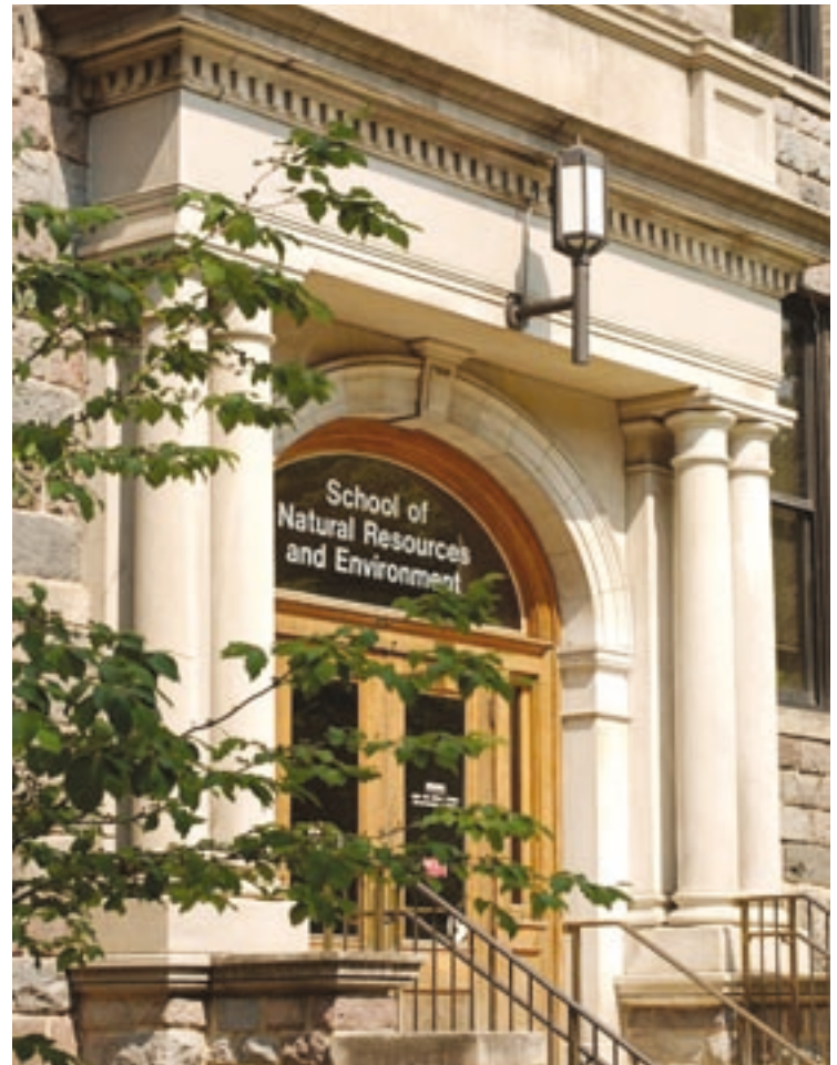
University of Michigan, Samuel T. Dana Building by William McDonough + Partners and Quinn Evans Architects, recipient of Gold LEED certification
