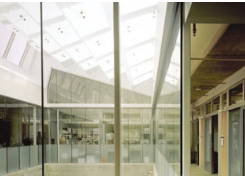
School of Nursing and Student Community Center University of Texas Health Science Center, BNIM Architects in collaboration with Lake Flato Architects.
