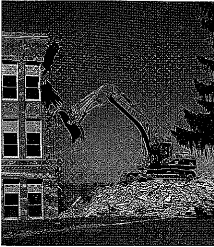
Fig. 5. The demolition of Normal High School, in Normal, Illinois, illustrates the volume of lost material that could have been saved if the building were reused. Courtesy of the Illinois Historic Preservation Agency.
