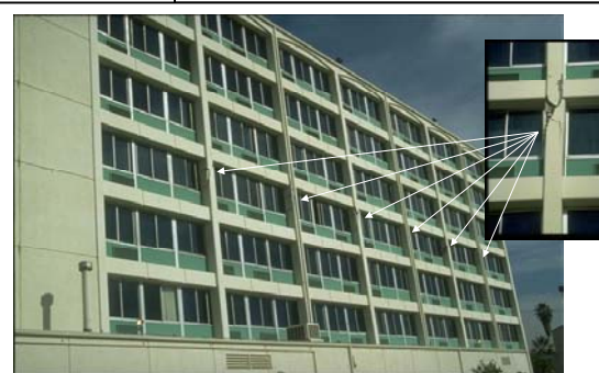
Figure 5 – Slab-column connection failure – Northridge earthquake
