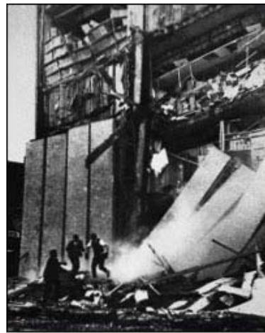
Figure 1. Concrete panels falling from the J.C. Penney store, 1964 Alaska earthquake.
