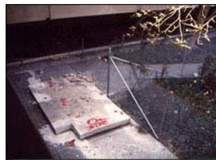
Figure 1. Concrete panels falling from the J.C. Penney store, 1964 Alaska earthquake.
