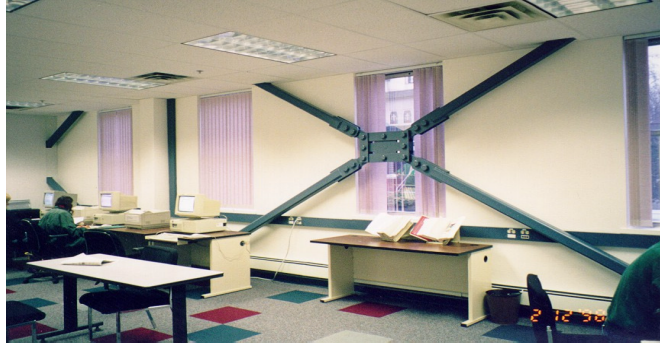
Figure 1 Harry Stevens building: X-braced friction damper
