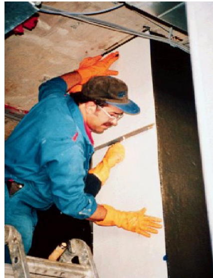
Figure 3 Port Alberni Building: CFRP application on a column
