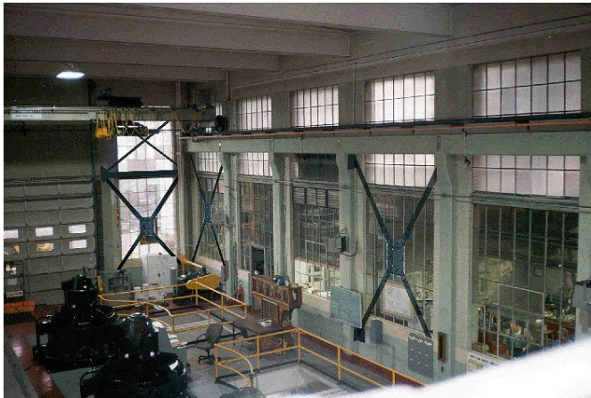
Figure 2 Pump House building: rendering of installation of friction dampers
