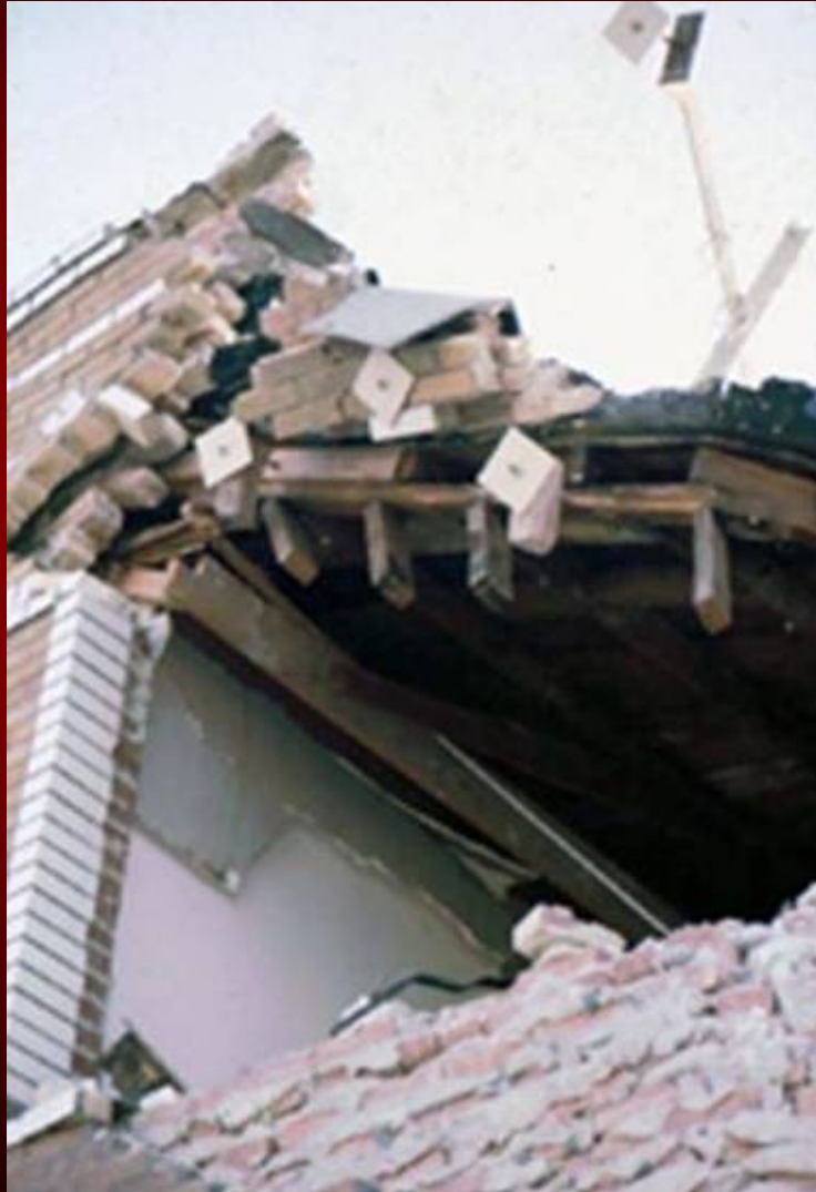
Corner failure
