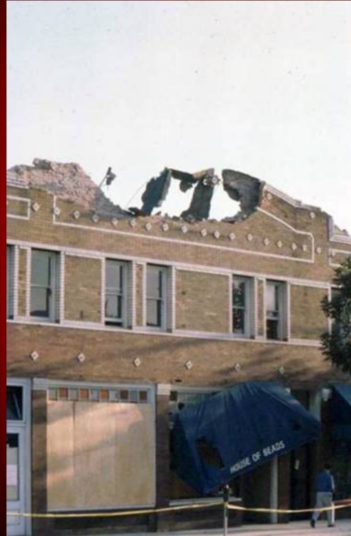
Parapet failure
