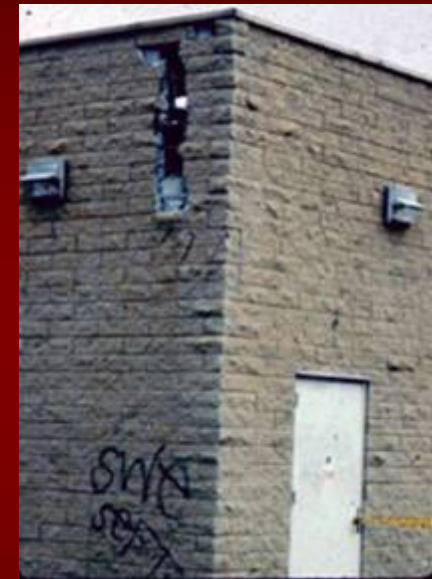
wall cracks
